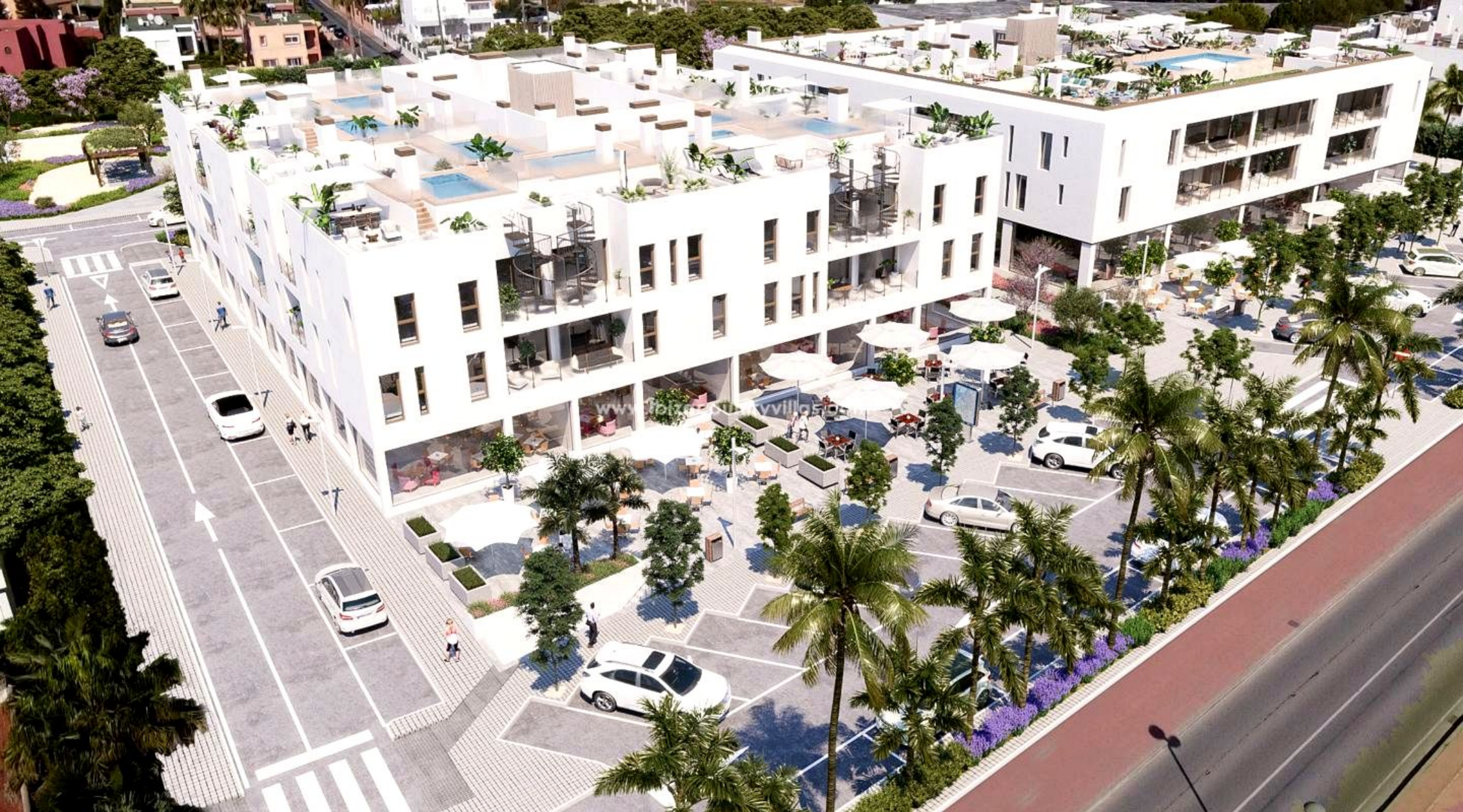
Building with 26 homes in the new Gavina development, featuring two and three-bedroom apartments, garage, commercial premises, and penthouses with private pool.
